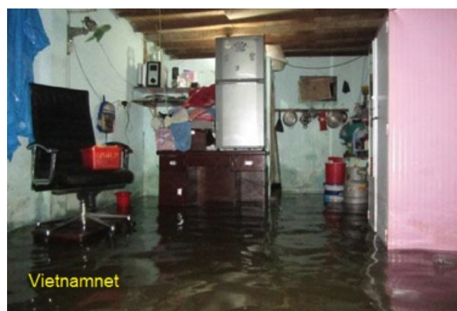
FIGURE 10 HOUSEHOLD FURNISHINGS RAISED OFF THE FLOOR TO PREVENT FLOOD DAMAGE
