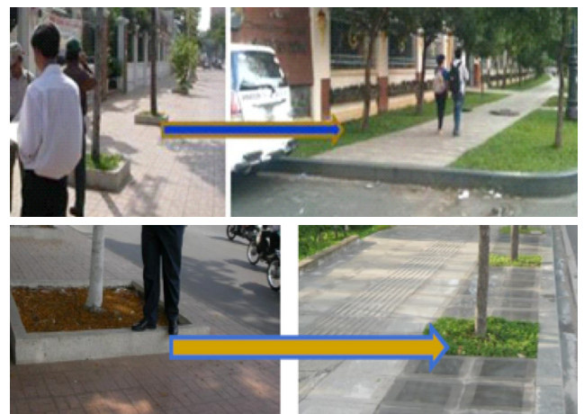
Improving water absorption of sidewalks (Truc, 2015)
