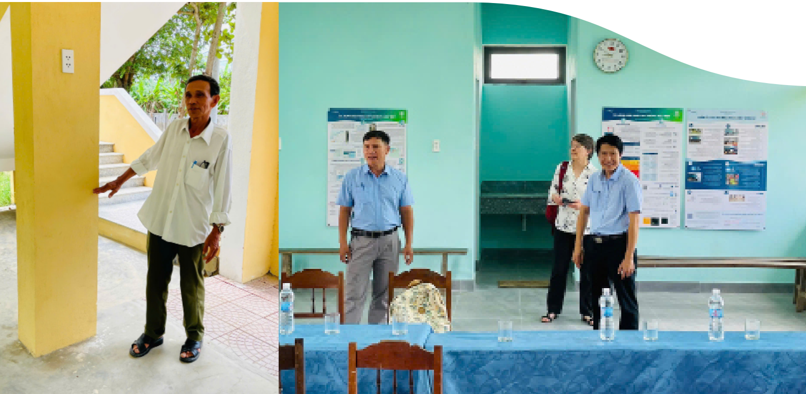
(Left) Flood level of the previous flood in the new shelter. (Right) Inside of the new shelter © Photo: Tho Nguyen, ISET Vietnam
