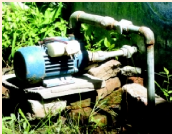
Pumping water from a supply main: Kathmandu
