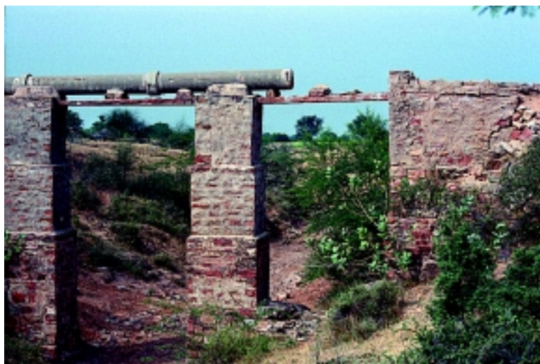
Supply line abandoned due to groundwater overdraft in Rajasthan
