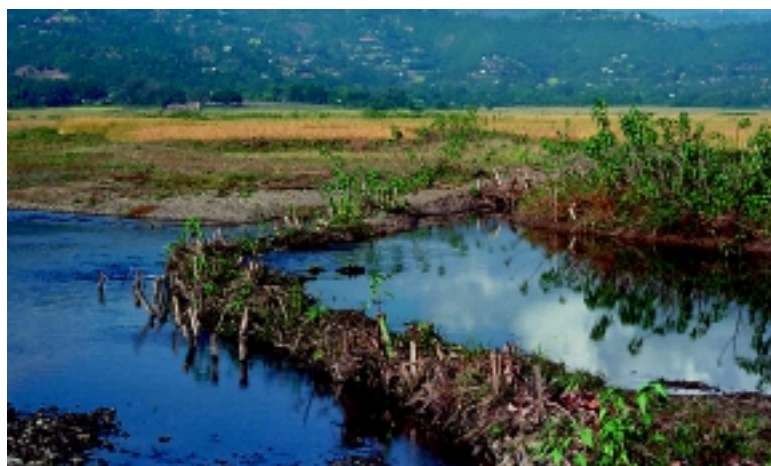
Irrigation parcels in Madi phaant use brushwood dam diversion
