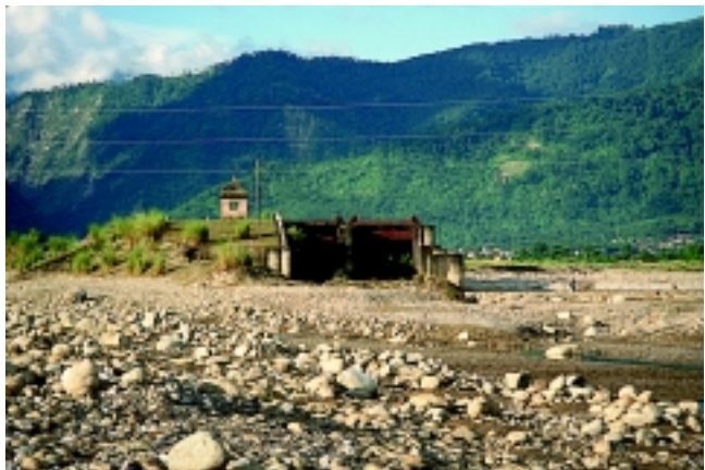
3 Abandoned Butwal barrage
