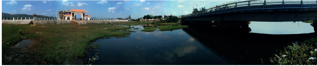
Photo 13. Quang Trung University blocks the flow of floodwater through New bridge on highway 19.
