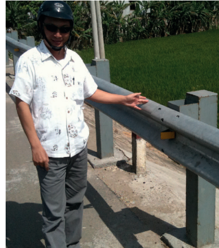
Photo 10. Height of floodwater on Highway 19.
