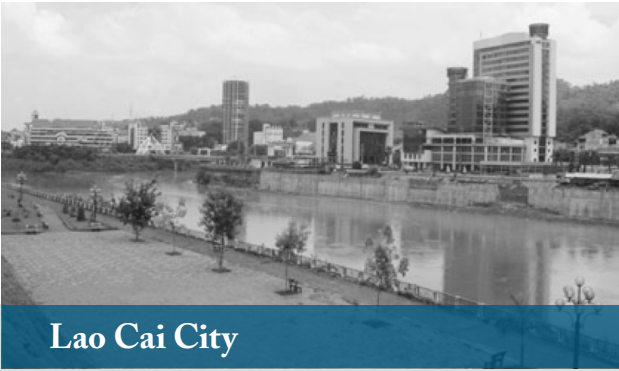
Image: A section of Red River embankment in Lao Cai City
